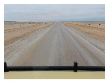
Here the roads or locally known as pads, are built with salt water. Driving on a salt made road is just like driving on a tared road. However, in case of rain it may all look different. These roads then can get very slippery and muddy.
